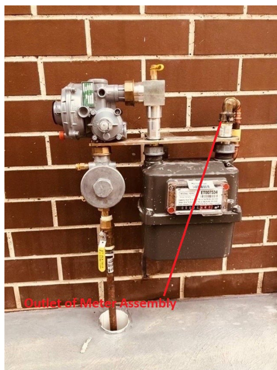
FIGURE E2 – Residential gas meter assembly – Model M10
