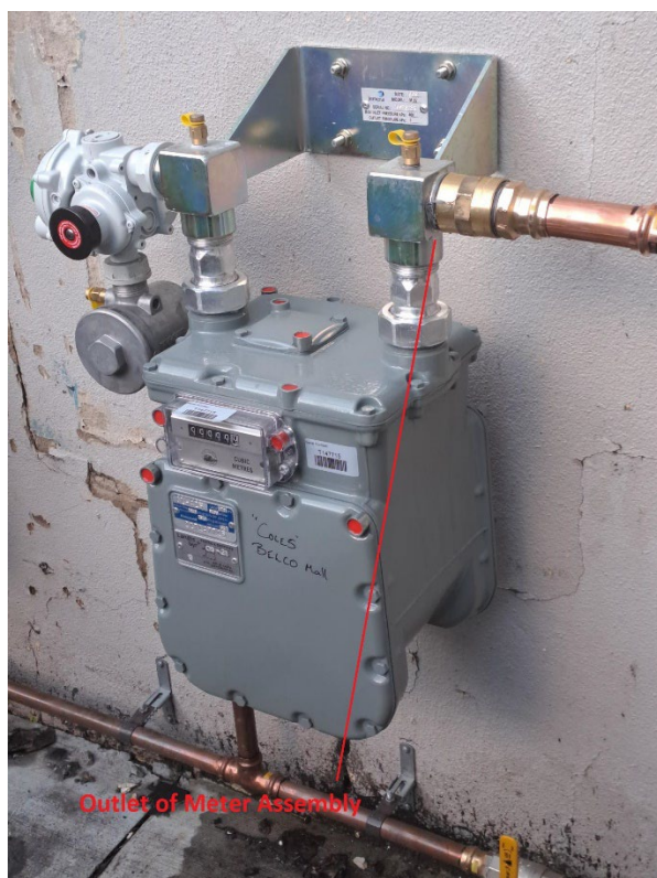
FIGURE E4 – Residential gas meter assembly – Model M25D
