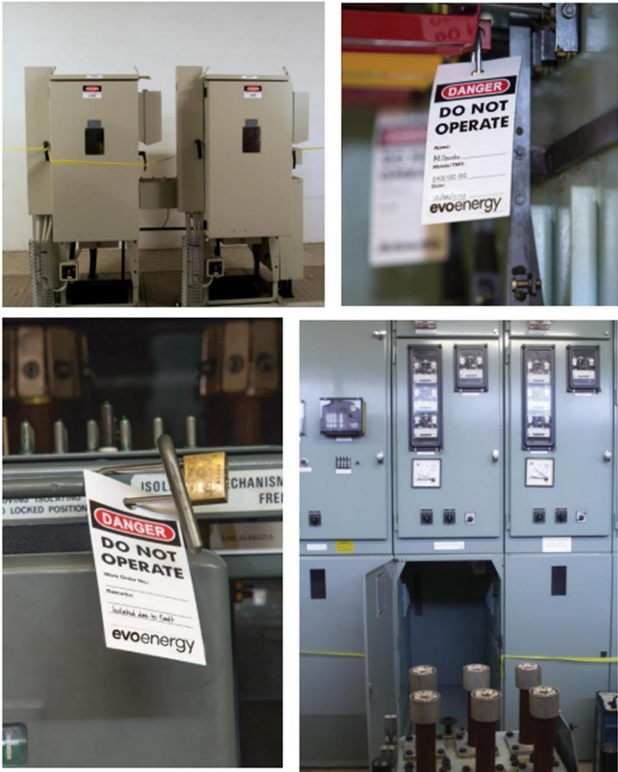
Figure 8. EXAMPLES OF VARIOUS HV APPARATUS WHICH IS TAPED AND/OR DANGER TAGGED TO CONTROL ACCESS TO VARIOUS PARTS OF THE APPARATUS
