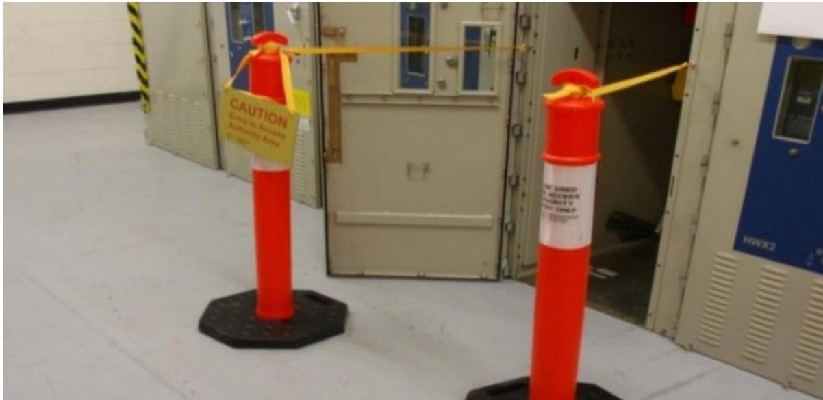
Figure 5. Example of switchgear under Access Authority with the Yellow Tape-In Method defining the entry area. Refer to Clause 7.7.4 Descriptions of barriers and signs for correct signage.
