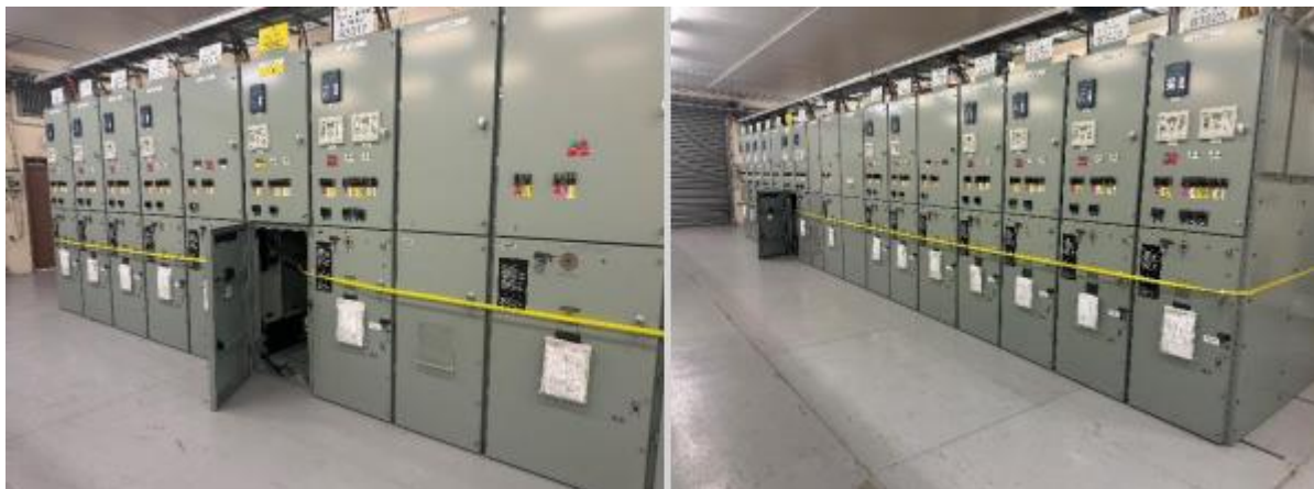
Figure 6. An example of the Yellow Tape-Out Method used on indoor metal-clad switchgear
