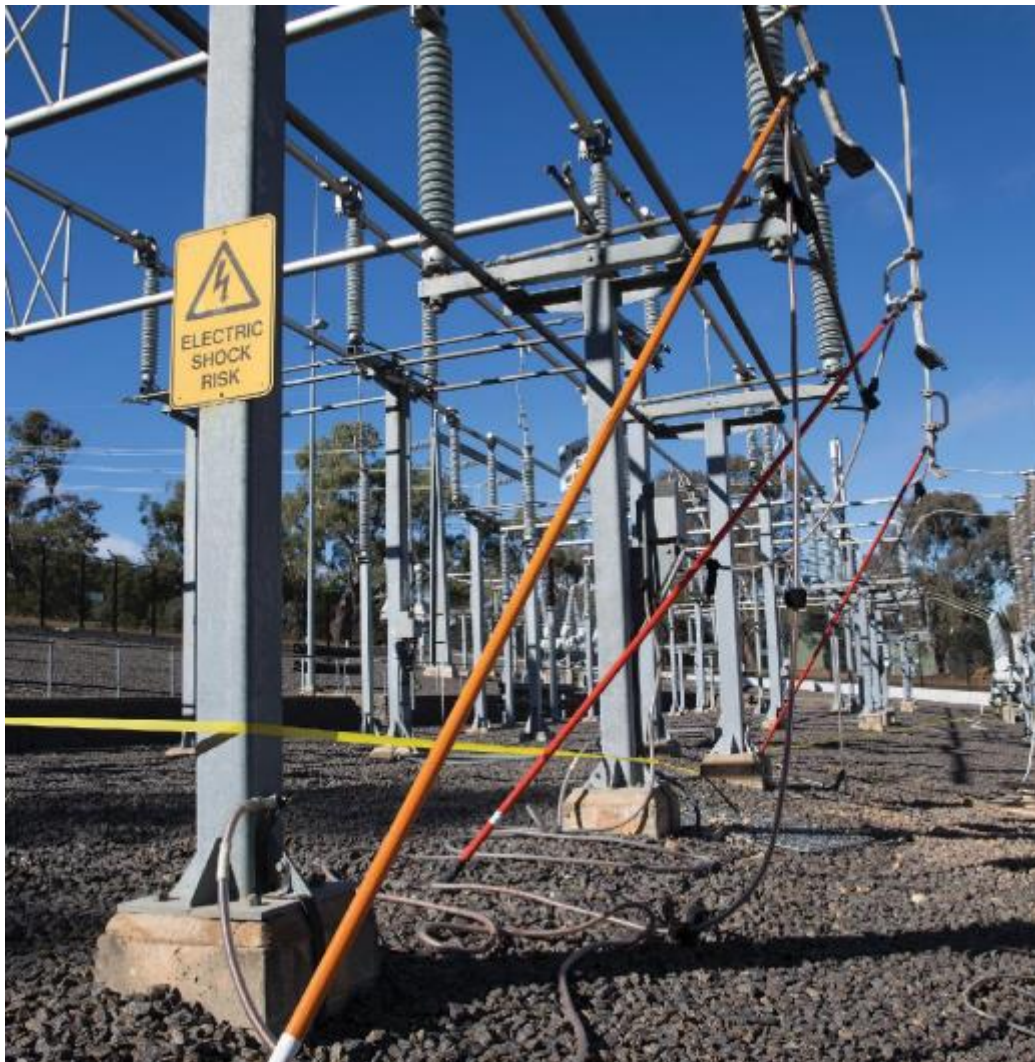
Figure 9. EXAMPLE OF OPERATIONAL EARTHS IN ZONE SUBSTATION
