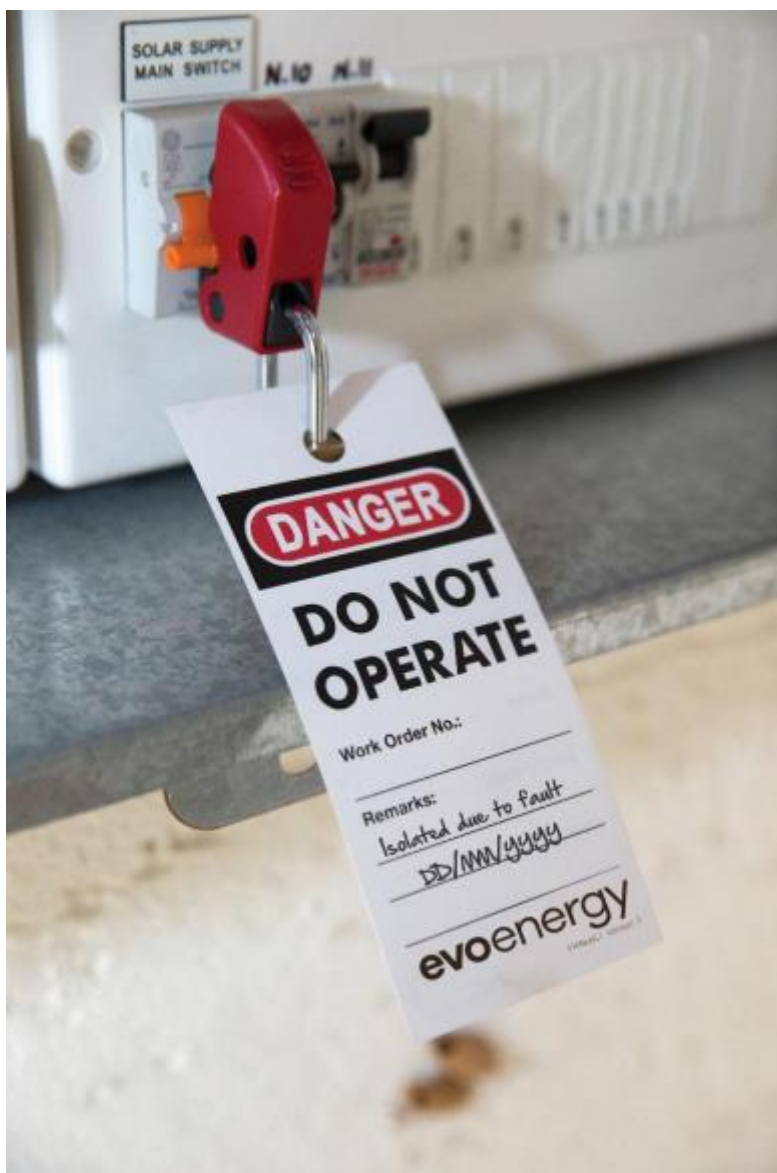
Figure 1. Example of 'Danger – Do Not Operate Tag'
