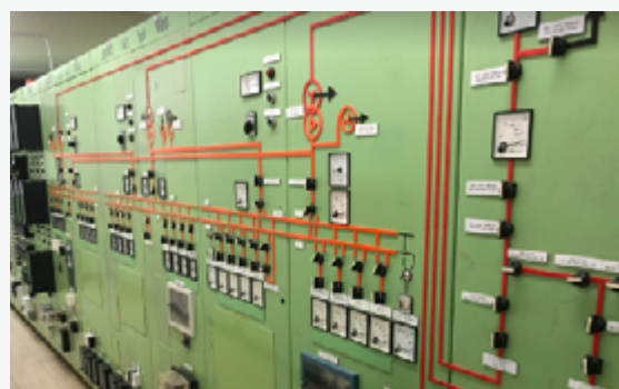
Figure 31. Wanniasa Zone Substation: 11kV Switchboards and Secondary Systems
