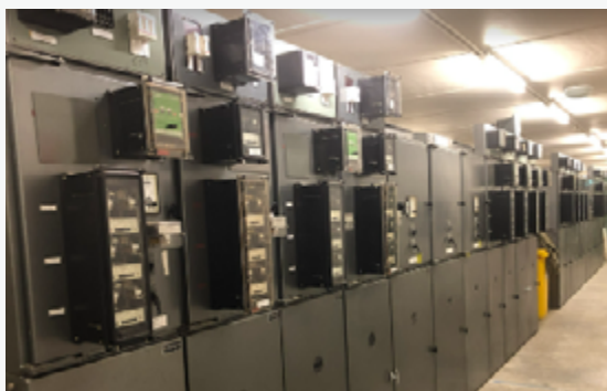
Figure 31. Wanniasa Zone Substation: 11kV Switchboards and Secondary Systems
