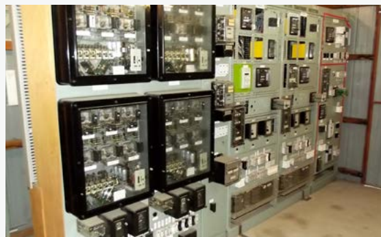
Figure 31. Fyshwick Zone Substation: Outdoor wooden pole strung busbars. Indoor 66kV electromechanical protection relays
