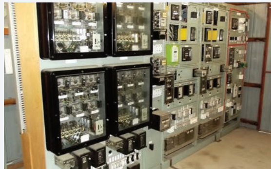
Figure 28. Fyshwick Zone Substation: Outdoor wooden pole strung busbars. Indoor 66 kV electromechanical protection relays
