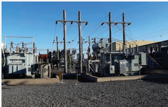
Figure 28. Fyshwick Zone Substation: Outdoor wooden pole strung busbars. Indoor 66 kV electromechanical protection relays
