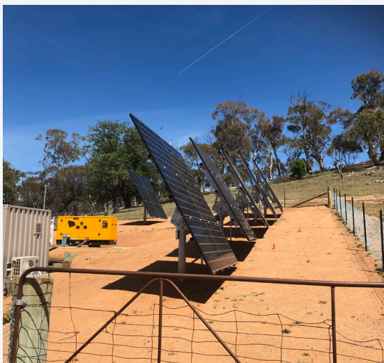
Photo: Gudgenby Homestead before and during RAPS installation
